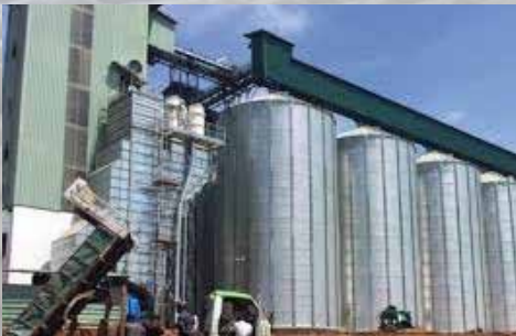
| Grain Warehousing and Logistics Components
