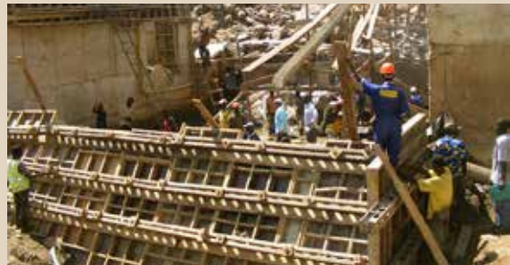
| Construction of Nyangak hydro power station
