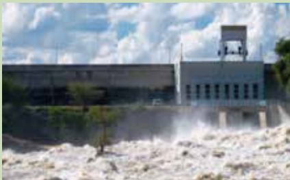
| Muzizi Hydropower station
