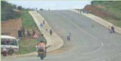
| Kaiso-Tonya Road, connecting to the oil fields
