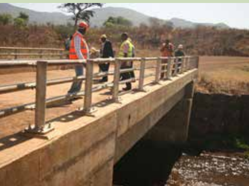
| Aringa Bridge in Lamwo
