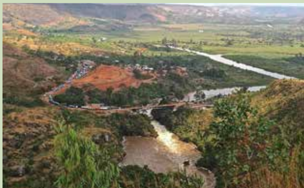
| Nyimur Multipurpose Water Resources Project
