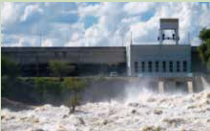
Muzizi Hydropower station
