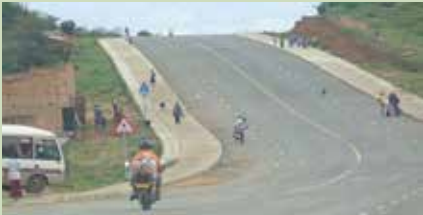
Kaiso-Tonya Road, connecting to the oil fields
